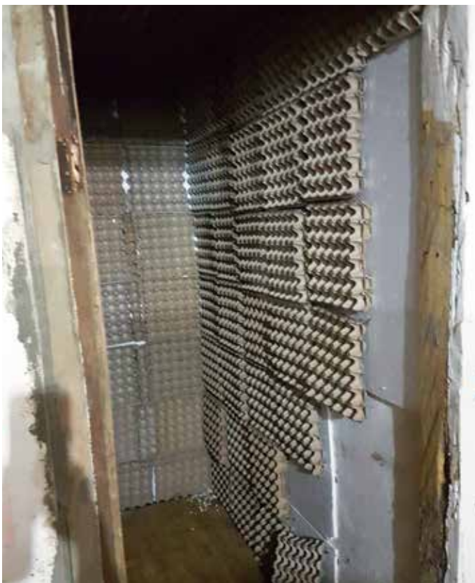
Makeshift audio studio lined with egg cartons 用鸡蛋盘筑成的临时录音室。
