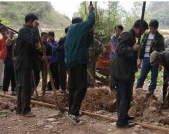
Villagers working together on the water project.
